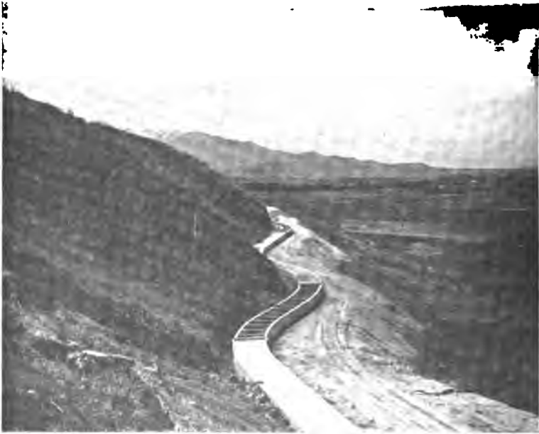
FIG. 162.—High Line Canal, Spanish Fork Valley, Utah, Covered to Protect against Land and Snow Slides.
